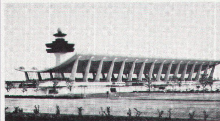
33 Dulles International Airport, Chantilly bei Washington, Virginia, USA, 1958–1962. Eero Saarinen and Associates
