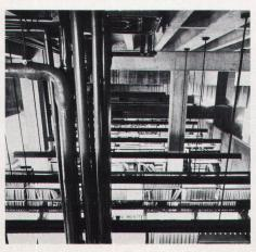
ble duct high velocity system). The offices are supplied with hot and cold water. Individual fan coil units thereupon produce the right air temperature in the offices. The separation between these two systems was made in the first instance for reasons of cost.
