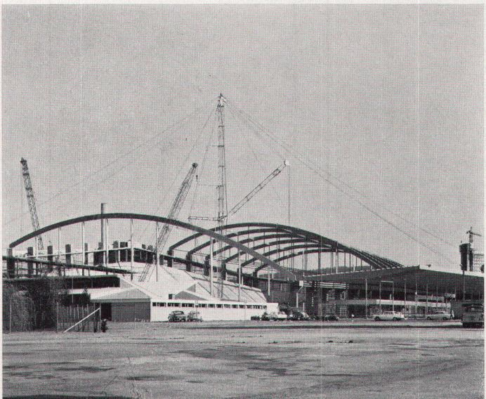
Thirteen trusses, glued-laminate double-jointed arches, span the ice surface and the grandstands of the Allmend rink in Berne. Tie rods of steel take up the horizontal stresses. The roof skin itself consists of translucent PVC corrugated plastic panels
