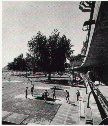
Strandbad Bellerive in Lausanne Avenue de Rhodanie 23 1936/37. Architekt: Marc Piccard BSA/SIA, Lausanne
