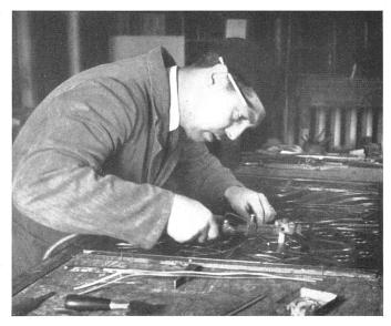
$11\ \ Verl\"{o}ten$  der Bundstellen | Le verrier soude les jointures | The glassmaker solders the joints
