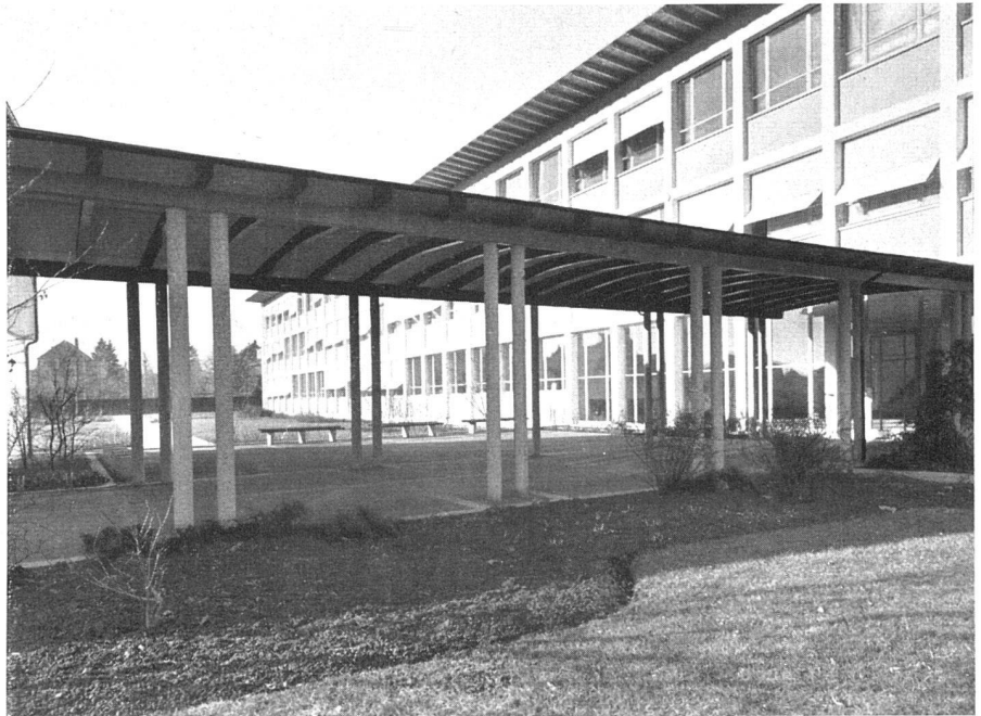
Pausenhalle und Klassentrakt | Préau couvert et aile des classes | Covered recreation area and main wing
