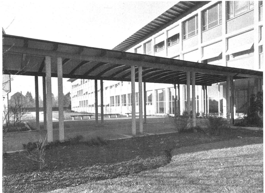
Pausenhalle und Klassentrakt | Préau couvert et aile des classes | Covered recreation area and main wing
