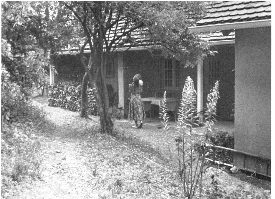
Blick in das Höfli von Westen / Vue sur la courette / View in the court from west
