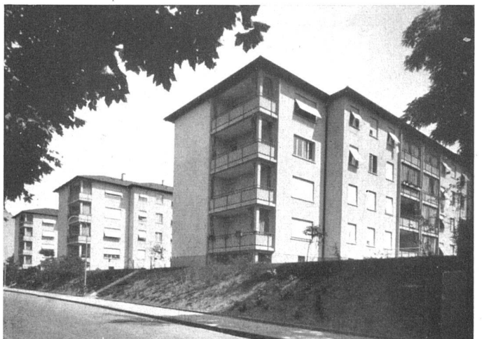
Nordwestansicht | Vue du nord-ouest | View to north-west
