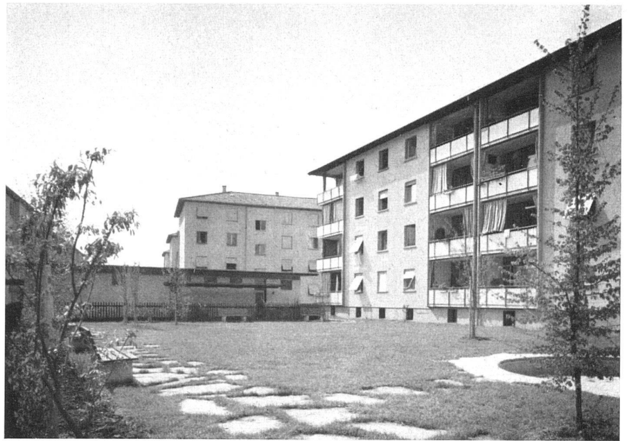
Ostansicht | Façade est | View to east
