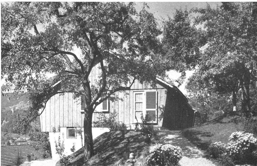
Ostansicht | Façade est | View to east
