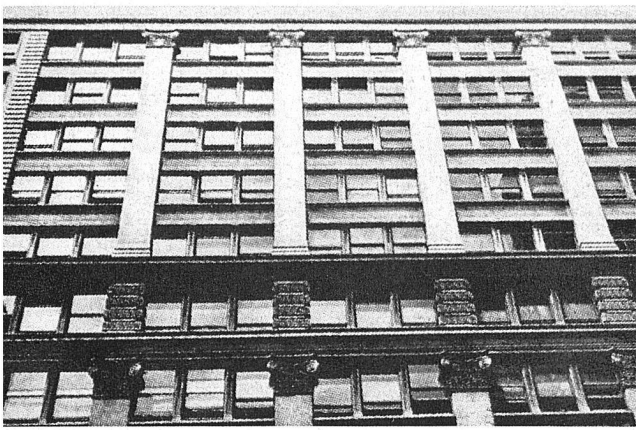
am Le Baron Jenney, Fair Building Chicago, 1891. Stahlskelettbau ebener Fassade
