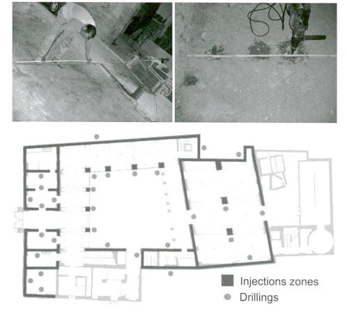
Fig. 2: Above: foundation survey at Palatium Vetus. Below: survey and intervention map.
