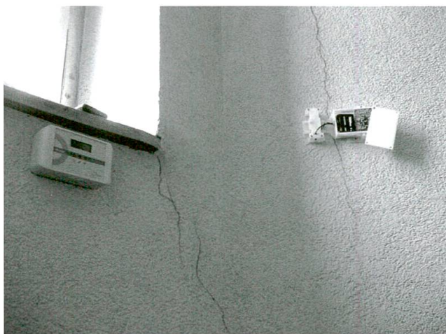
Fig. 15: Easy Crack Monitor System®.
