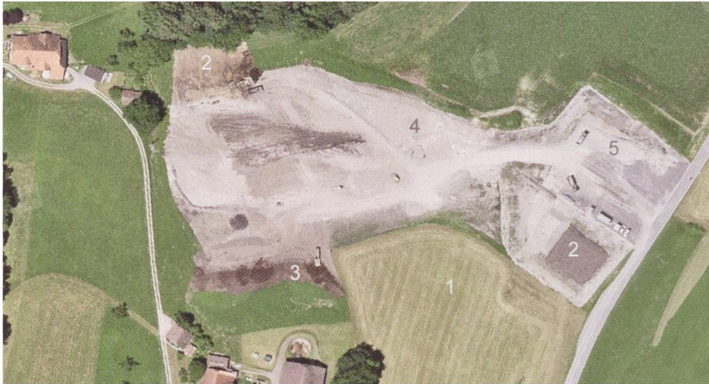
Abb. 1.2 c: Bauschuttdeponie Eyacher. Stand 2019.
