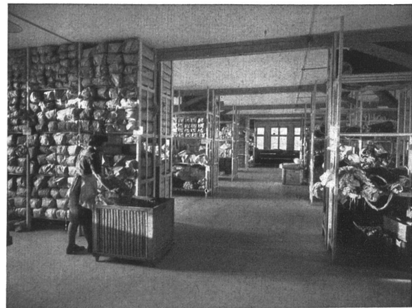
Stores department. — Almacén.
