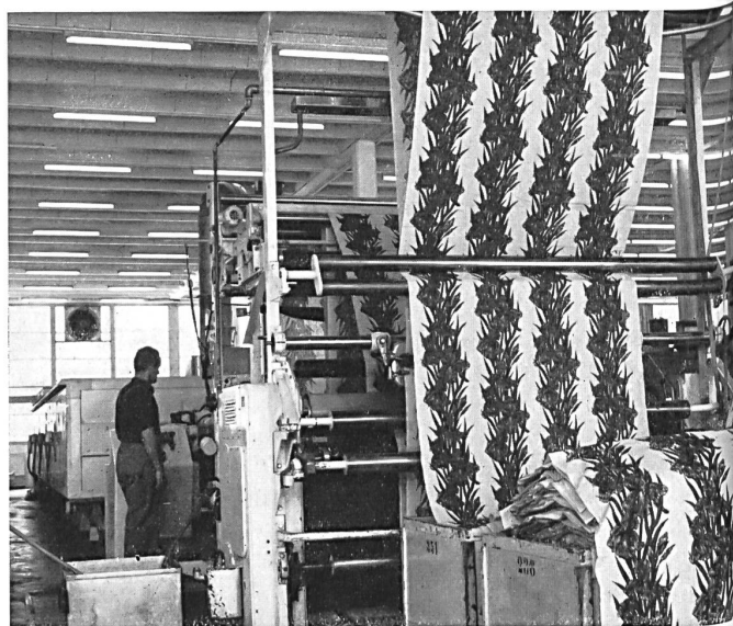
Fabric starting off in a dressing machine
