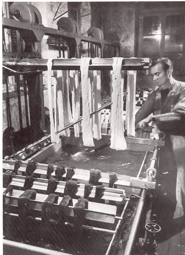
Hank dyeing machine for silk twists.
