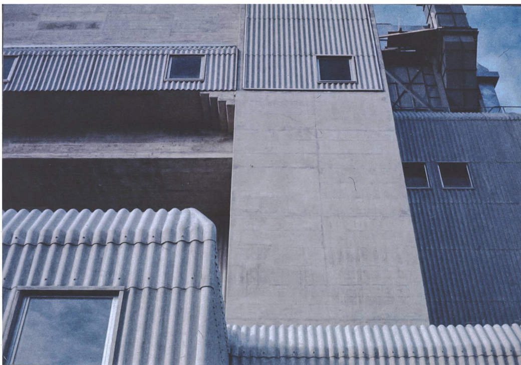
KVA Linth, Niederurnen GL, 1966–1973. Façade detail, 1973. Image: gta Archives / ETH Zurich, Pierre Zoelly
