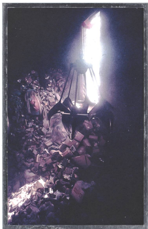
KVA Linth, Niederurnen GL, 1966–1973. Waste bunker with grappler, 1973. Image: gta Archives / ETH Zurich, Pierre Zoelly
