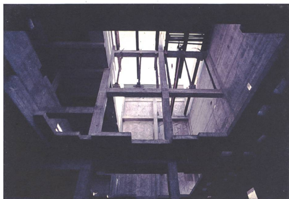
KEZO, Hinwil ZH, 1966–1976 (2 phases). Construction process, 1975. Image: gta Archives / ETH Zurich, Pierre Zoelly
