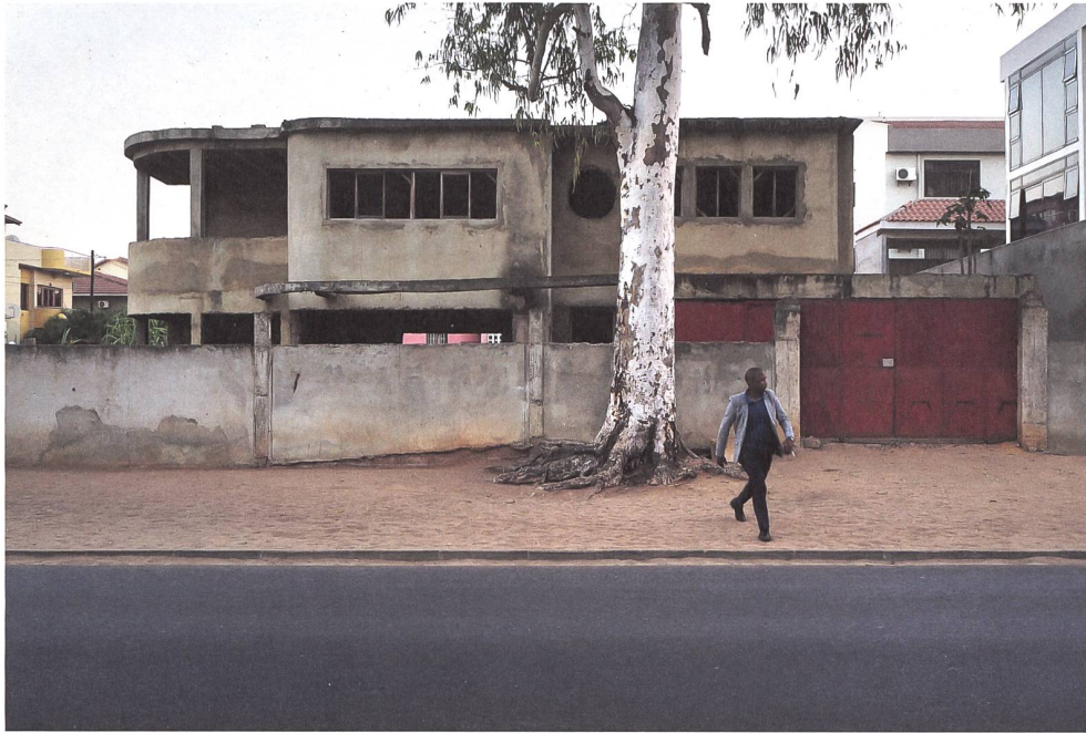
(Fig. 1) Construction site in Polana Caniço, Maputo, Mozambique, 2019. Photography: Silvia Balzan
