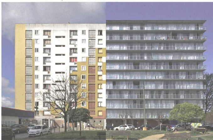
fig. g Transformation of buildings G, H, I, Grand Parc, Bordeaux, France by Lacaton & Vassal, Druot, Hutin, 2016 © Philippe Ruault
