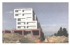
The building is constructed with precast concrete elements in three shades of pink, carpentry is made of champagne-coloured anodized aluminium. From our perspective, this first element shows the scale and the orientation of the future campus, using colours which allude to Auguste Perret's buildings located on the other side of the campus; to our client and many politicians, it appeared in a very different way. In their eyes, it was a very serious visual
