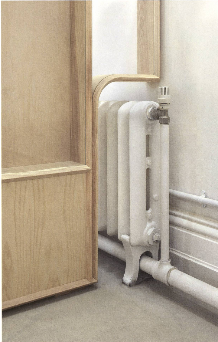
fig. g jumping over the radiator, ground floor studio partitions
