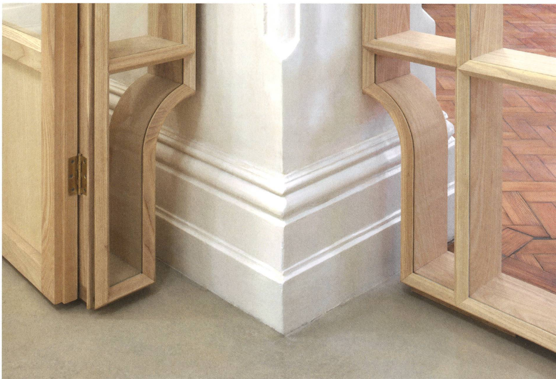
fig.f curved detail, ground floor studio partitions
