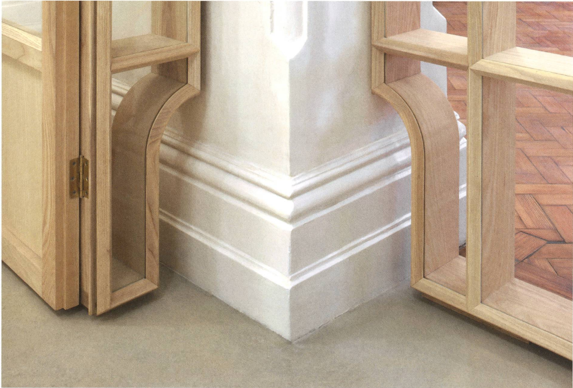
fig.f curved detail, ground floor studio partitions
