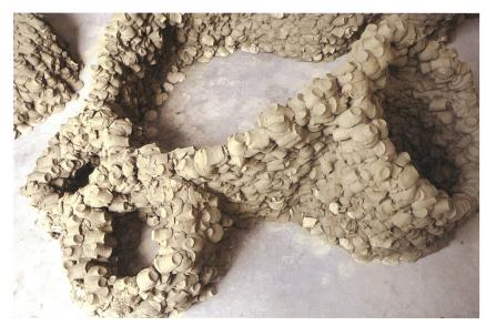
fig. d Detail of the final structure with deformed clay projectiles forming the wall texture. Photograph: Yves Roth.
