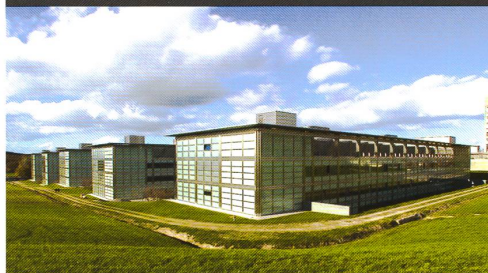
ETH Hönggerberg, 2. Phase, Zürich
