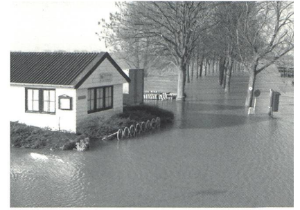
Flood of the Wal river in Holland, Photo by Ch. Giroit, 1995
