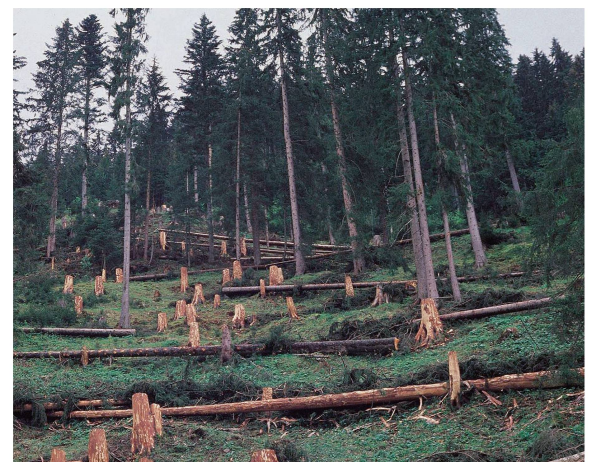
Fig 9 Rockfall protection by obstacles consisting of logs positioned on the slope (Photo: Bernhard Maier).
