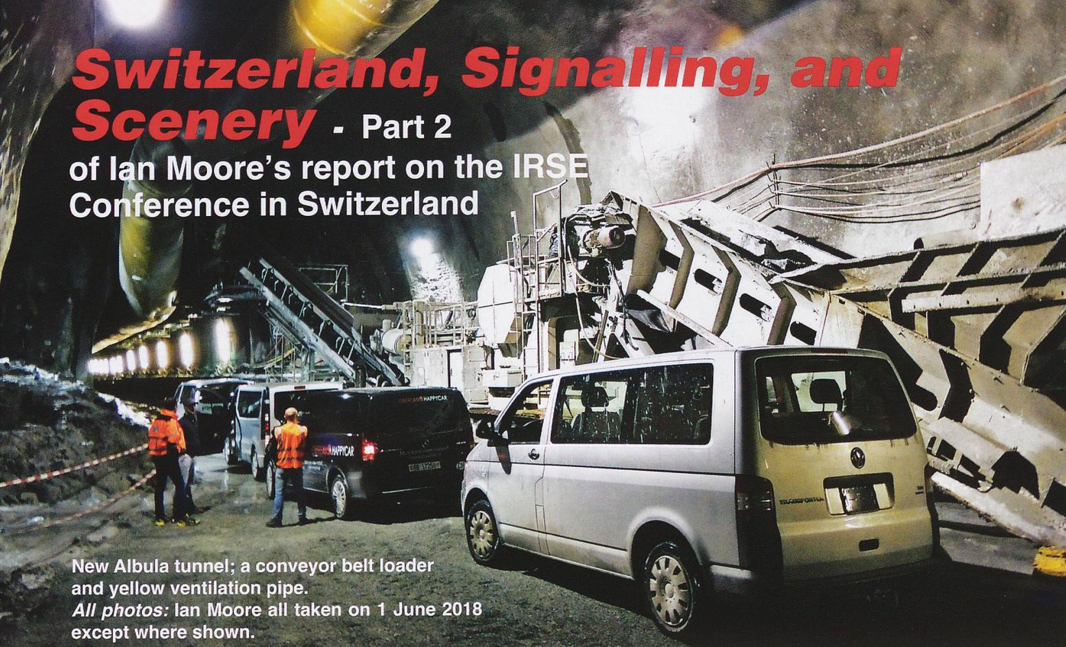
New Albula tunnel; a conveyor belt loader and yellow ventilation pipe.
