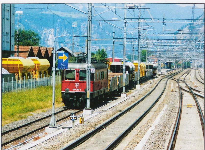
Approaching Altdorf from the south. ERTMS Block Marker (virtual signal), and shunt signal to the left and a balises pair to the right.
