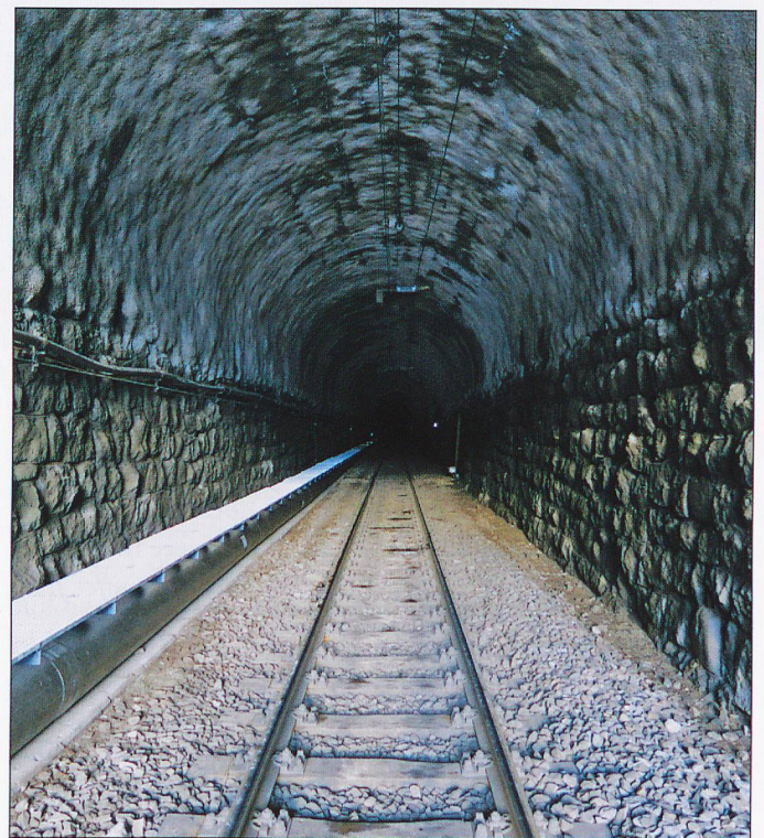
Inside the existing Albula Tunnel – Wikimedia.
