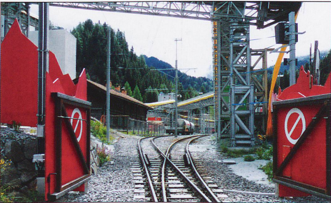
Preda facing south and east of the station.
