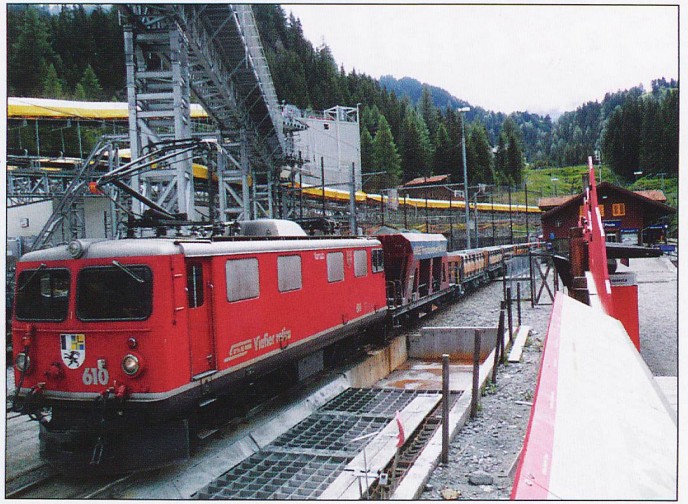
RhB Ge 4/4 No.610 on tunnel construction duty in June 2018.
