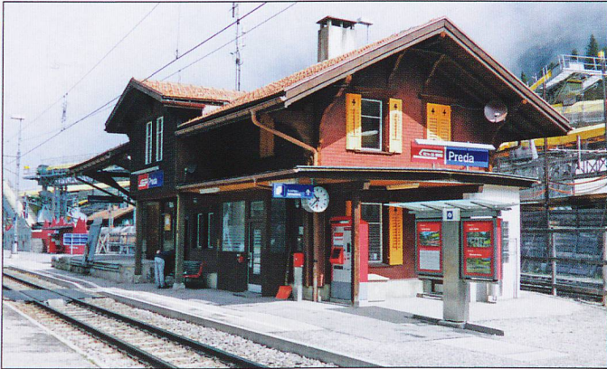
Preda in 2018 with the construction site backdrop to the east side.
