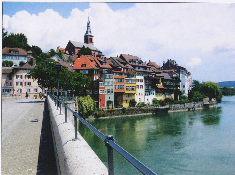
Border bridge at Laufenburg, towards Germany/Apfelkuchen.
