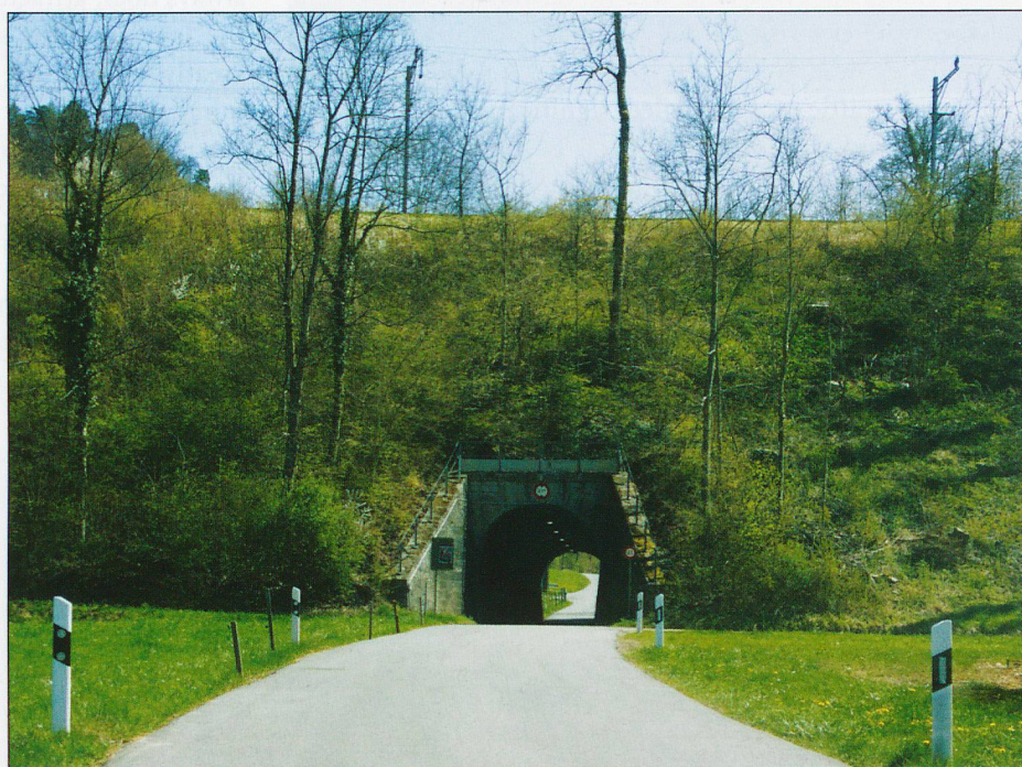
TOP: Sissach: 1854 Lineside cottage. RIGHT: Sommerau: the old main line climbing at 23 ‰ on a massive embankment above a local road.
