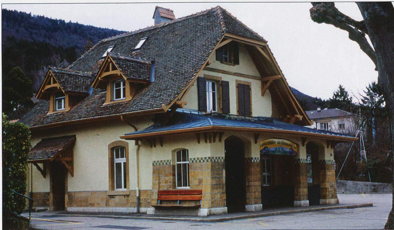
La Coudre Lower station, a substantial building.
