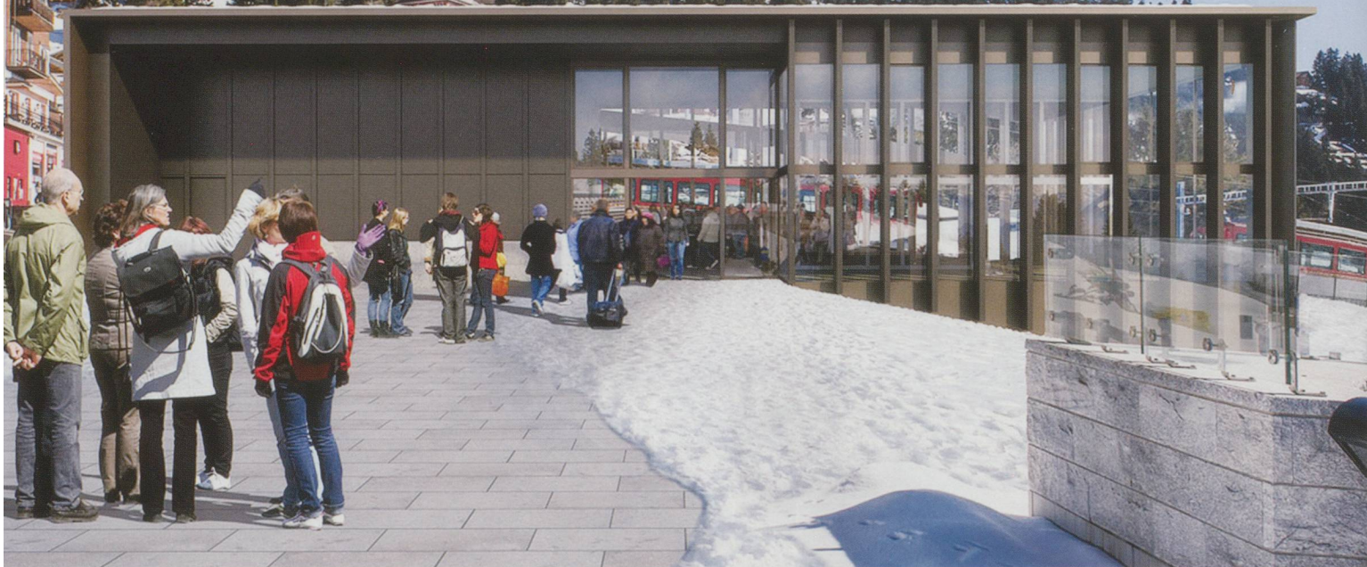
The new building at Rigi Kaltbad.
