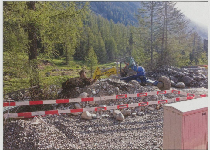
Preparation work for the new Albula tunnel at Spinas.
