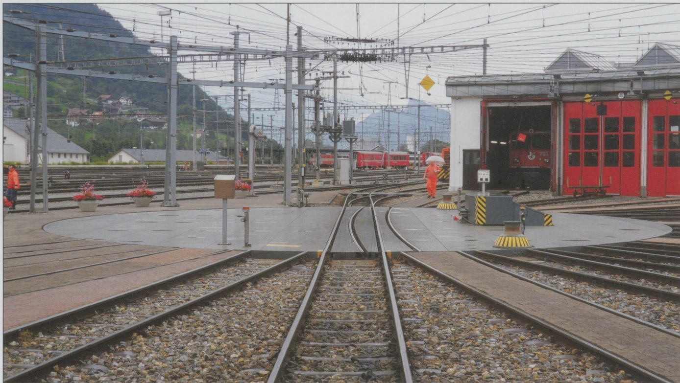
The distinctive turntable in the works.
