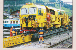
Unloading a track maintenance machine at Zweisimmen from the standard to meter gauge. PHOTO: Roy Marriott
