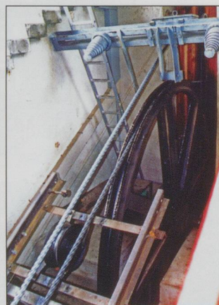
BELOW: Sonloup Funicular winding gear
