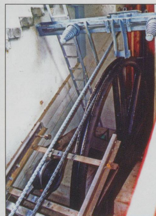
BELOW: Sonloup Funicular winding gear
