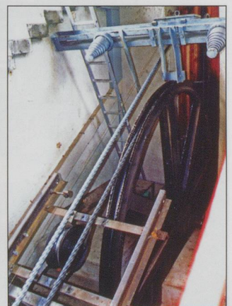
BELOW: Sonloup Funicular winding gear
