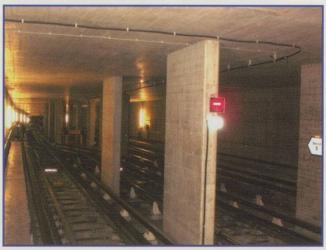
A1:8 incline, and an 80m radius curve, start right at the end of a station. Platform doors are on the left.
