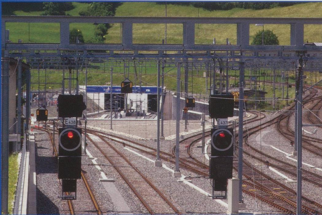
the old “mountain” route. Presently, the heaviest trains using the Lötschberg Base Tunnel have a hauled load of 3250 tonnes and a length of 750 metres. Freight trains will travel through the base tunnel at speeds up to 100km/h. Passenger trains will travel around 200km/h and, when fully
