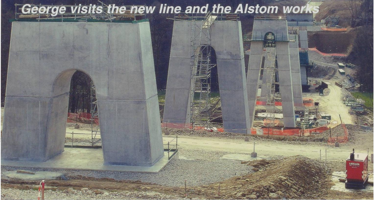
*These pillars are for one of the spectacular viaducts that will carry the line straight across a valley. Although the trains themselves are not that heavy, the pillars receive such a pounding from the 200 mph speed, they have to be this massive.*
