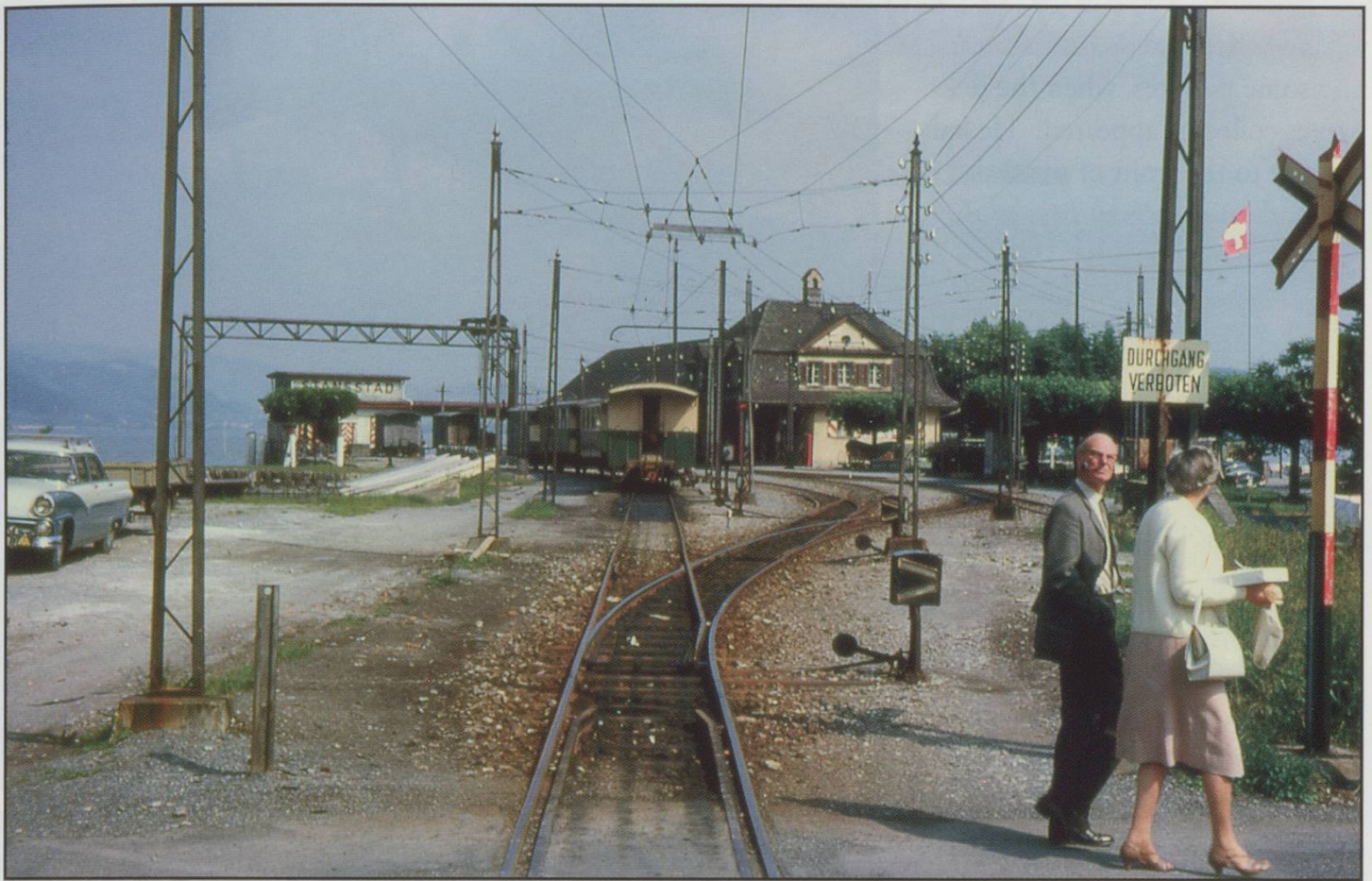
ABOVE: The old line crossing the road into the Harbour Station and the complication of the 3-phase wiring. NEXT PAGE, UPPER: Loco waiting to giving rack assistance. CENTRE: New bridge partially built looking towards the tunnel in 1964. LOWER: Timber false work for the high-level bridge under construction in 1963.
