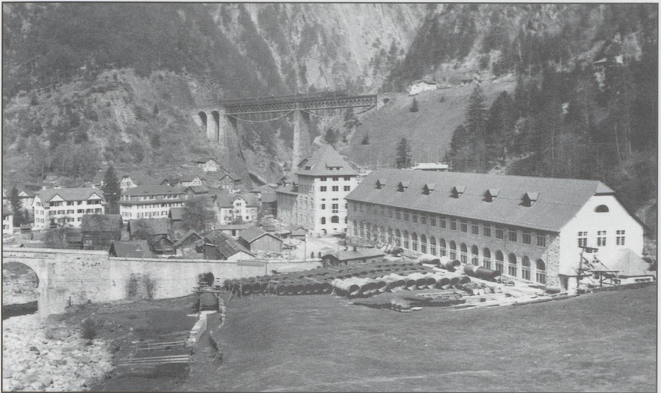
Amsteg. Power station.
