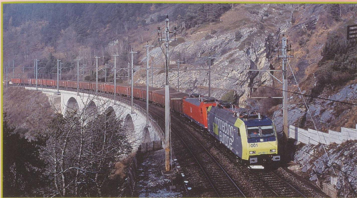
Co-operation in freight on the bls. One of the new bls 485 locos double hauls with a DB twin over the Lötschberg.
