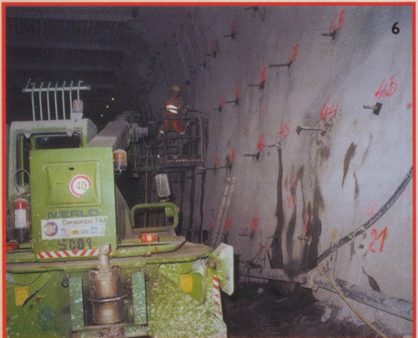
Photo No. 6: If all is well, the last set of reinforcements is fitted. These are the so-called anchors: they are long rods cemented into the surface of the rock, which help to hold back the reinforcement plates seen in photo 4, which are now behind a cement coating.
