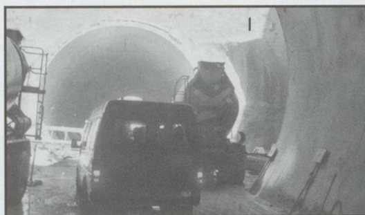
1. Inside the Zimmerberg tunnel, the cement lorry drives onto the loading platform, where it is fixed with chains.
