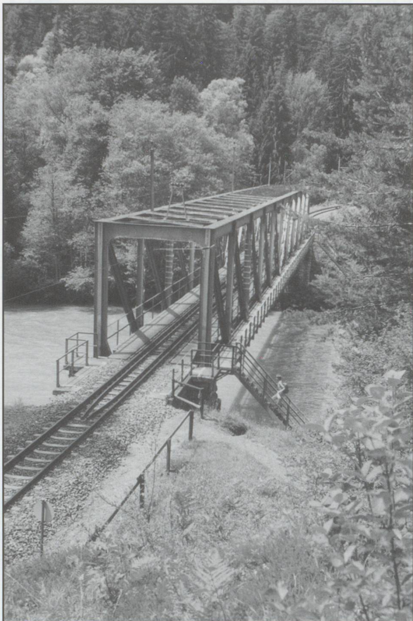
Bridge over (Kwai) Rhine below Conn, near Versam. 1.7.97. Photo: Pete Dyson
