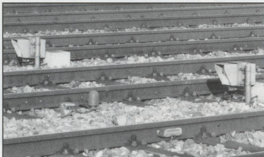
Muttenz. Feb. 2003. Wagon speed detectors, 1 per track.
