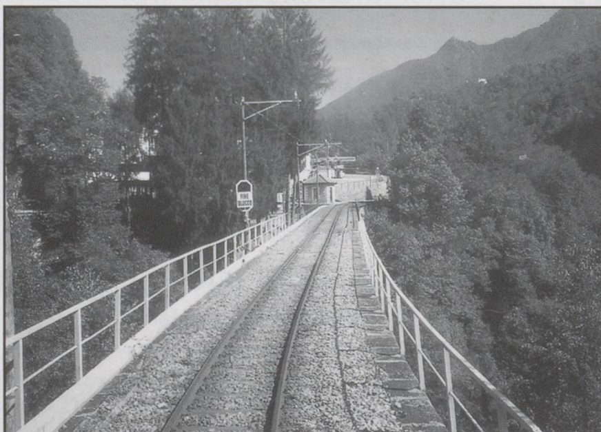
The viaduct at Camedo. 7/9/2000. Photo: Douglas Ellison
