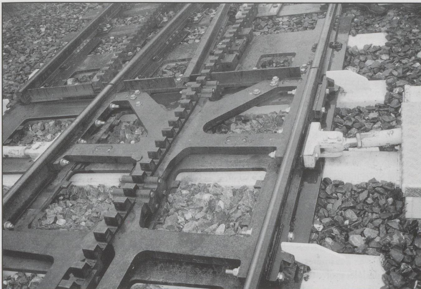
*The actual ends of the turnout in detail, the track really is straight through. To the left the diverging track can be seen partially intertwined with the straight route.*
