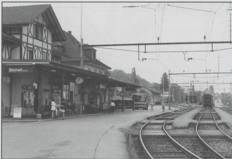
*Beinwil in August 1997. LH line was the branch platform. Wagons from the branch are stored in the centre road. Nowadays the RH loop is a truncated siding and wagons are left there, and the further centre road is the main line. A PTT Setra 315 awaits Beromünster passengers from the connecting train. All photos in the article are by Ernie Brack.*
