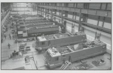
are completed and laid out in the area ready for the arrival of the body from the contractor. Locomotive bodies are in the main built by SLM Winterthur and shipped to Oerlikon on
