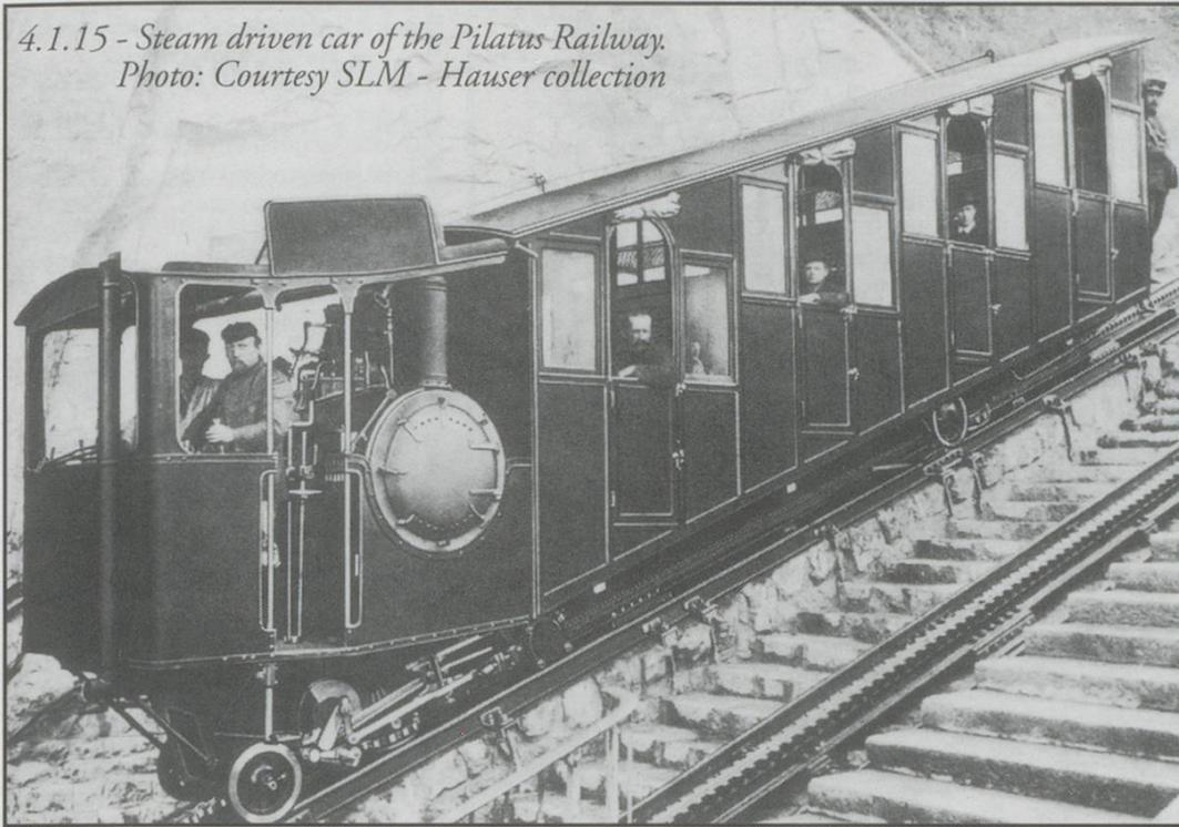
ing. 11 were supplied in 1887, a further 3 in 1888/9 and one each in 1900 and 1909. Designed as two axle vehicles, the downhill axle carried the machinery (boiler, drive mechanism, cab etc), whereas the passenger compartment was borne by the uphill axle. The seats of the latter are arranged in steps to compensate for the steep incline. The drive is shown in drawing 4.1.14. (see also photo 4.1.15 and technical data 4.1.16).
